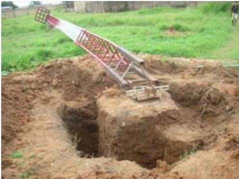
Shifting the large mass of concrete to get the tilt base level and secure was made difficult by all the rain.
